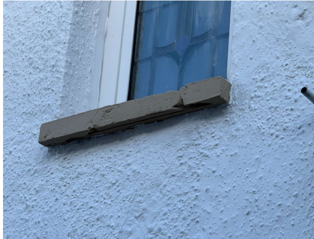
Damaged sill.
