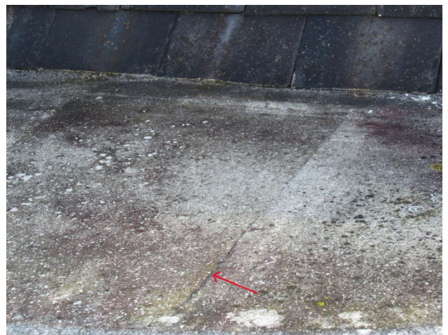
Hairline cracking.
