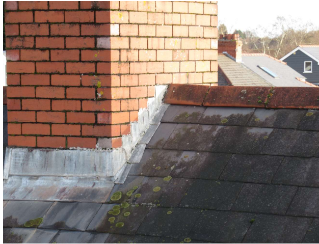
Note repair to lead.
