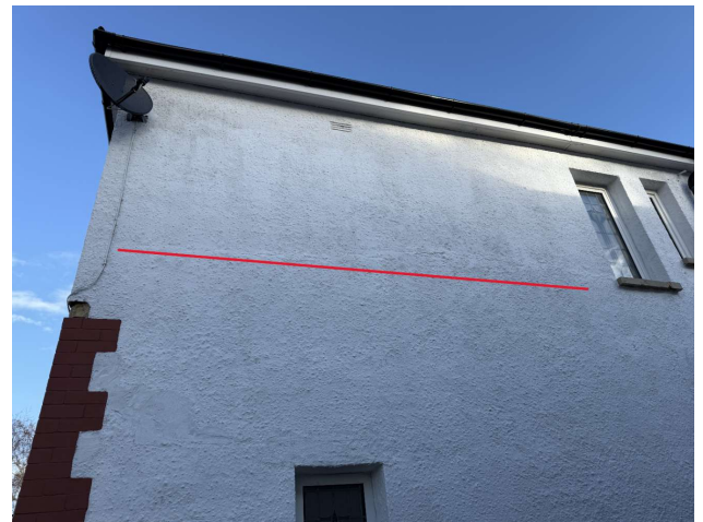
Horizontal cracking.
